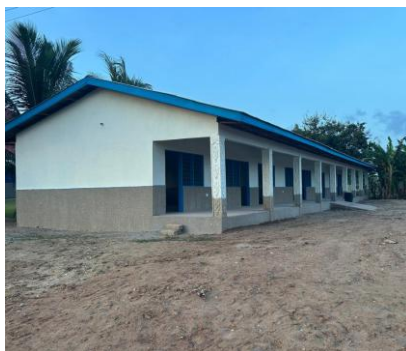
Junior High School building is nearly complete!
