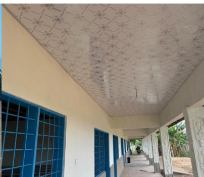
Finishing touches on the JHS building
